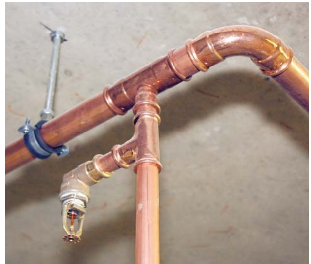
Fig. 10. Examples of low-pressure watermist pipes and fittings.
